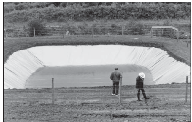
Figure 2. Elevated earthen reservoir with woven polyethylene liner
