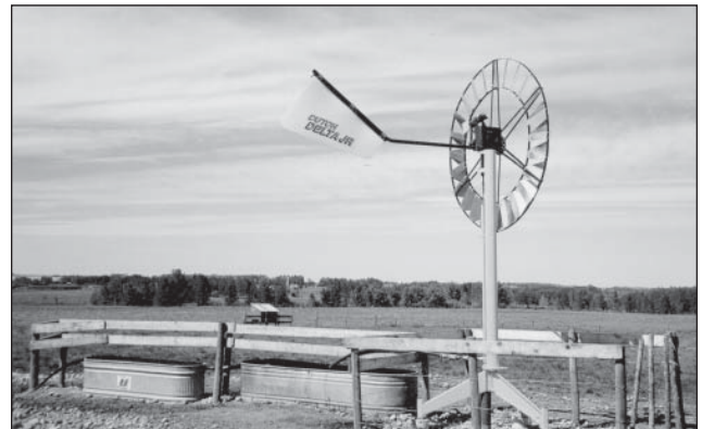
Figure 7. Wind-powered pumping system
